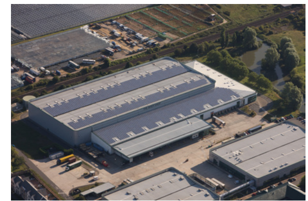
THE LARGEST SELF-FUNDED SOLAR PANEL PROJECT IN THE UK, AT OUR WATERSMEAD SITE IN LITTLEHAMPTON.
